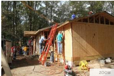
Volunteers from First Baptist Church work to restore a longtime vacant house from the ground up on California Street, north of Tennessee Street, where Gary and Josephine Montgomery will live. The Montgomerys, who direct a family ministry, hope their move brings a positive influence on children in the area. / First Baptist Church/Special to the Democrat
